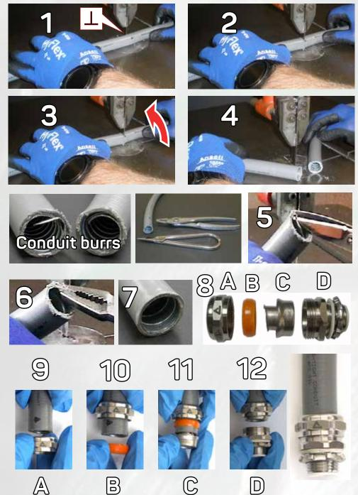
**NOTE**: ANACONDA SEALTITE<sup>®</sup> fittings for metallic conduit have similar parts, but the Food Grade compact fitting has different seals.
